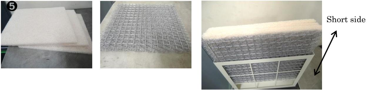
After inspection and withdrawing the filters and demister
